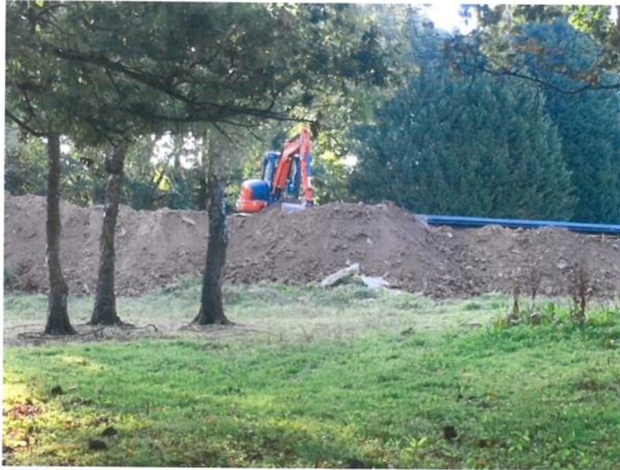
Photos of site at time of excavation works when earth bank to road was removed
